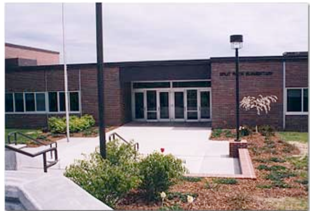
Split Rock Elementary
